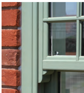
Run through sash horns
