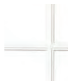
Georgian bars (fitted between panes of glass)
